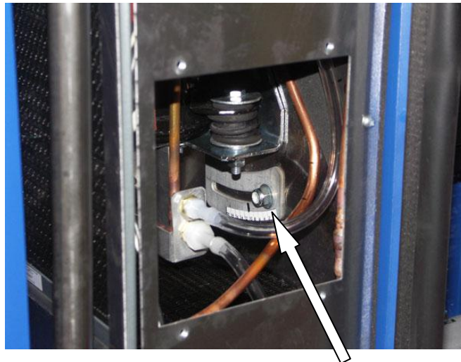
Loosen to adjust compressor
